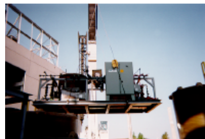
Convenient skid mounting for easy and cost effective installation .
